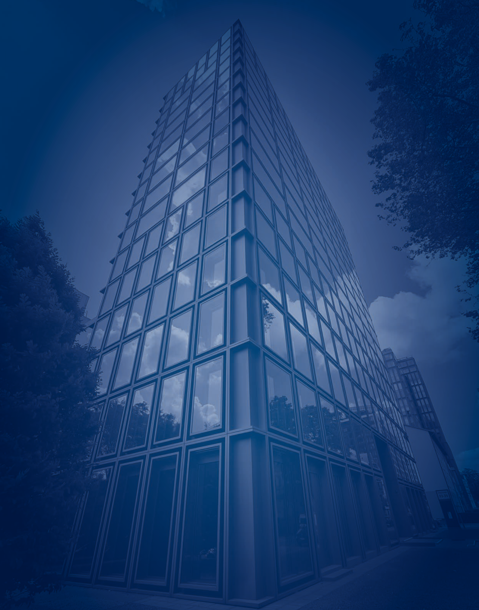
The Office of Lloyd Fonds AG in Frankfurt at "Ulmenstraße 23-25".
